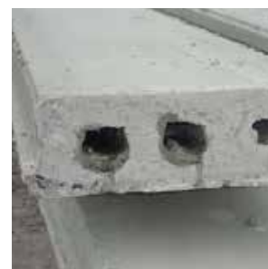
Prefabricated concrete plate + plaster
