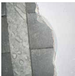
Concrete beam & block + plaster
